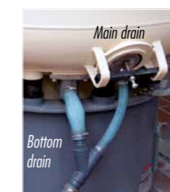
Combined media unload plug with effluent drain (main drain)
